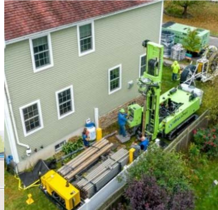
“Water Source” AKA geothermal or ground loop
